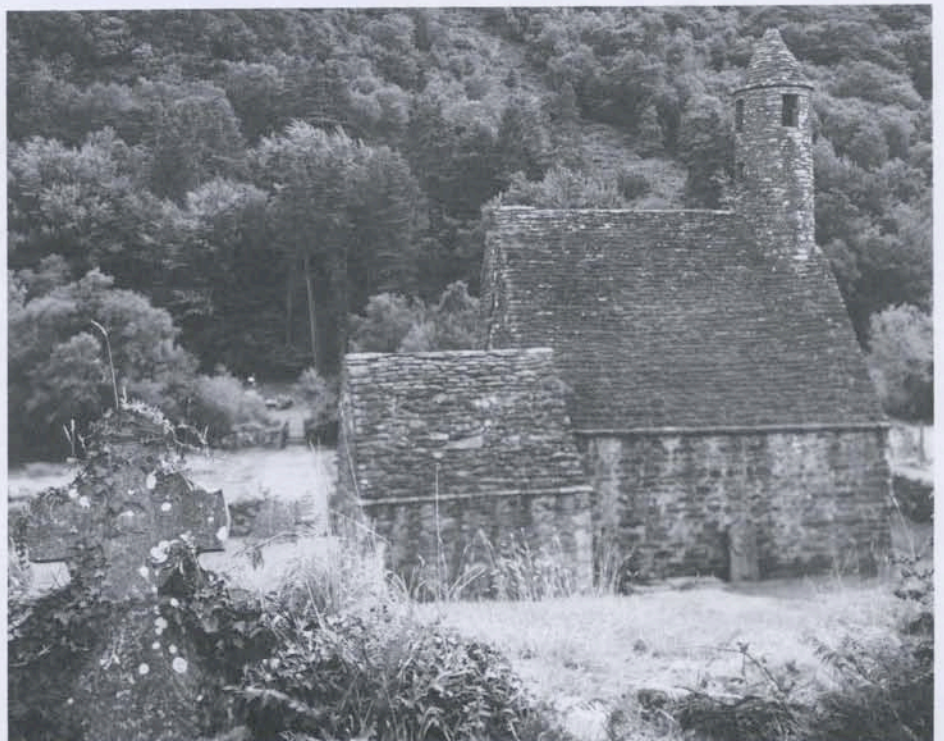
Saint Kevin's Church Cir. 6th c. Glendalough, County Wicklow, Ireland Corbeled stone roof and a belfry in the shape of a miniature round tower
