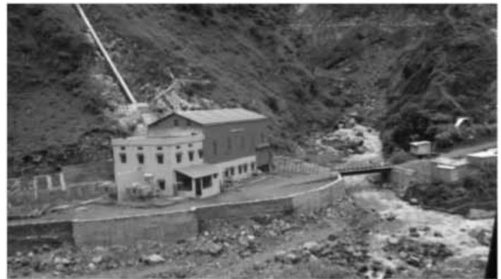
**Figure 1.** typical small scale hydroelectric production facility located in Chattrarri, Himachal Pradesh, India. Note visible penstock left of the building, and the discharge, not visible in the picture, at the bottom near the stream.
