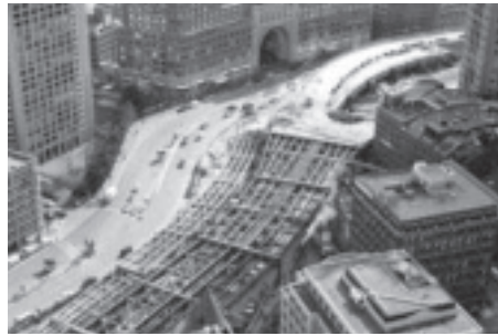
February 2004: An aerial view of the old elevated Central Artery (I-93) without its road deck just north of Rowes Wharf.
