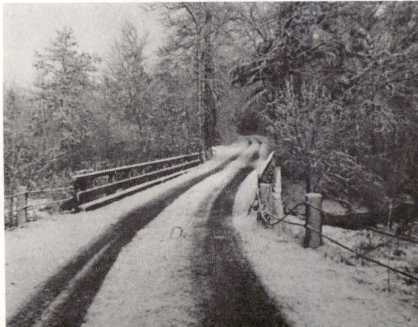
The Auburn Street bridge the morning after a snow storm.
