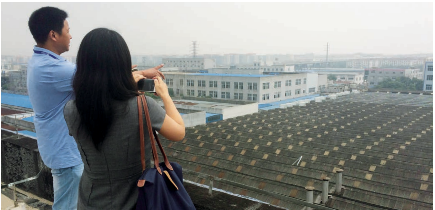
Distributed PV System on the Roof of an Industrial Plant, Changzhou. Author's photo.
